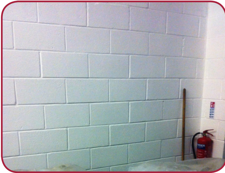
Glazecoat S.P. applied to Thermal Blocks
