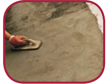
Rapid Set-Polymer Patch Repair
